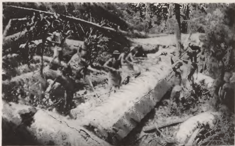
FIG. 4—"Squaring" mahogany logs in the bush. The man at the left with the two "machetes" is beating the time, and the men on opposite sides of the log are supposed to work in unison
